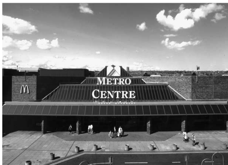
Figure 1: MetroCentre regional shopping centre, Gateshead
