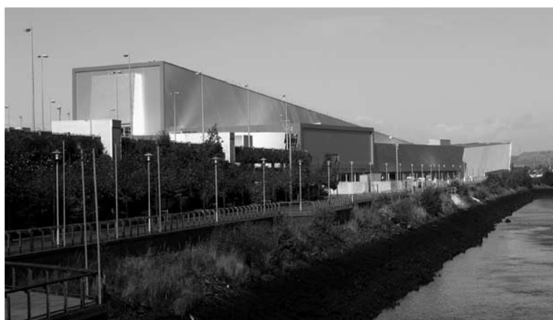
Figure 2: Braehead Shopping Centre, Renfrewshire
